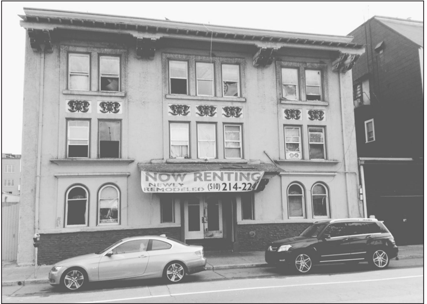
The West Grand Hotel has been sued by the Oakland City Attorney for slum conditions and dangerous code violations.
